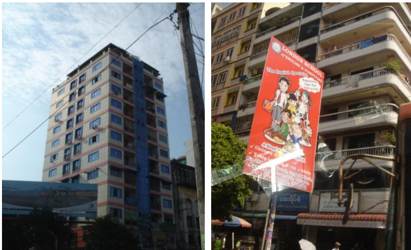
Photos: Typical new apartment buildings in Yangon (May 2013)
